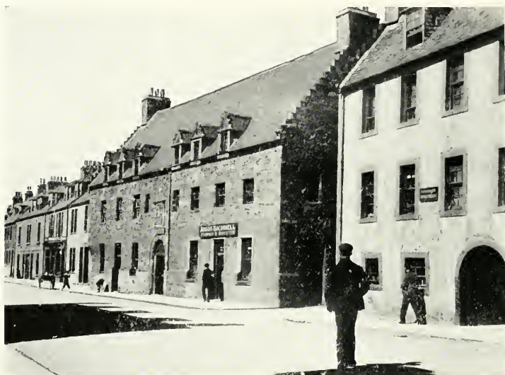
OLD HOUSES IN CHURCH (KIRK) STREET, INVERNESS
