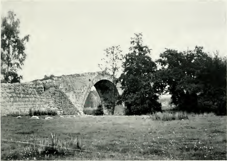
SLUGGAN BRIDGE OVER THE DULNAIN NEAR INVERLAIDNAN, WADE'S MILITARY ROAD
