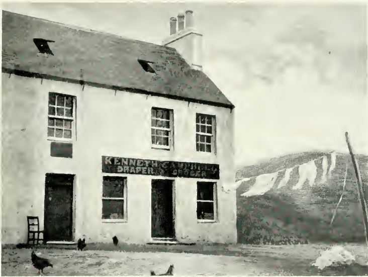
House at Scalpa, built on the site of the one in which the Prince stayed when on the island. A stone tablet over the door commemorates the fact. Vide note 1, p. 207.
